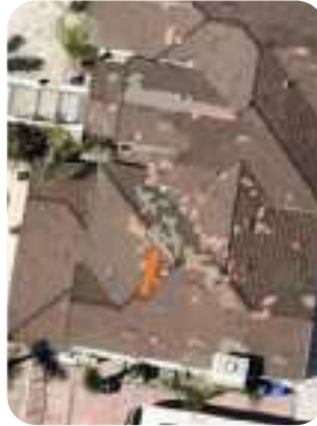
Missing Shingles
